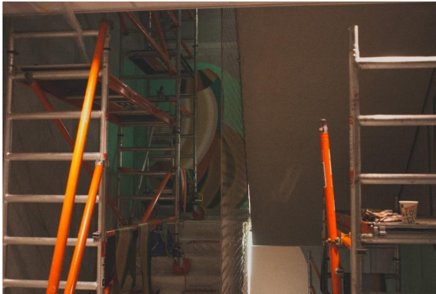
image i. Mural under construction.
